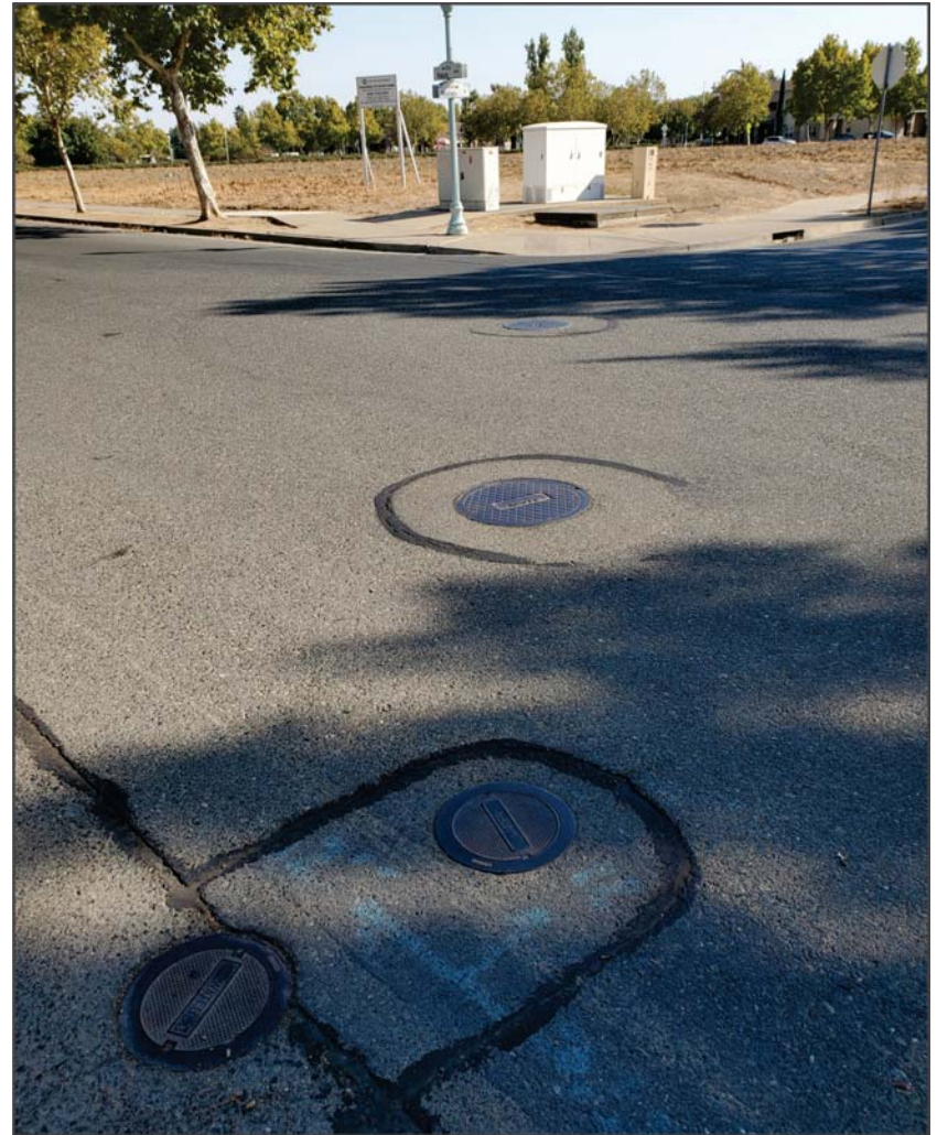
Photo 11: Various utilities within Vaux Avenue which runs along the north property boundary.
